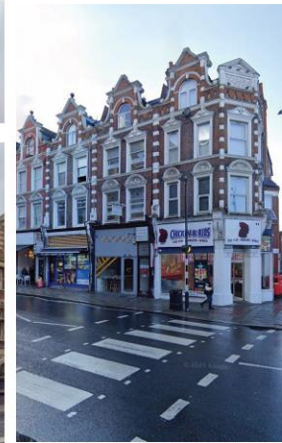
Image of Tottenham Lane high street
